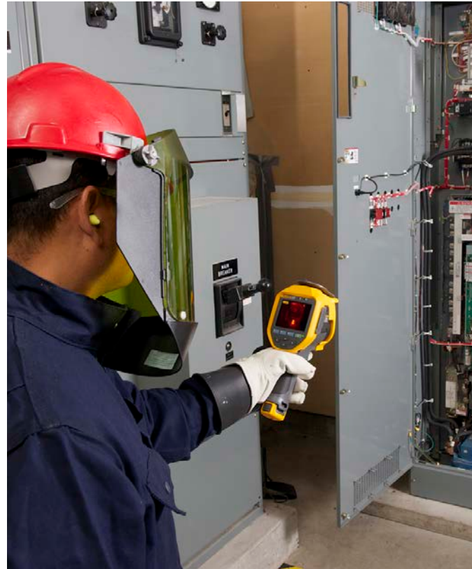
When scanning a live electrical panel, wear appropriate 70E personal protective equipment for arc flash and stand at least four feet away.
